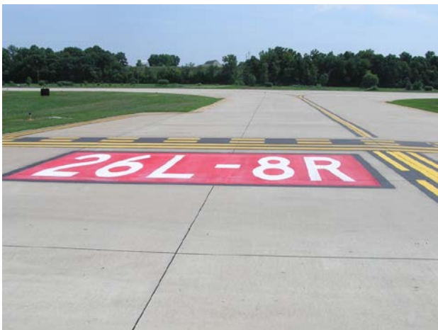
Figure 8c : Surface Painted Hold Position Sign
