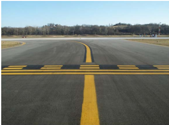
(Figure 6) Hold Short Lines and Taxiway Centerline
