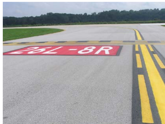
Figure 8d : Surface Painted Hold Position Sign
